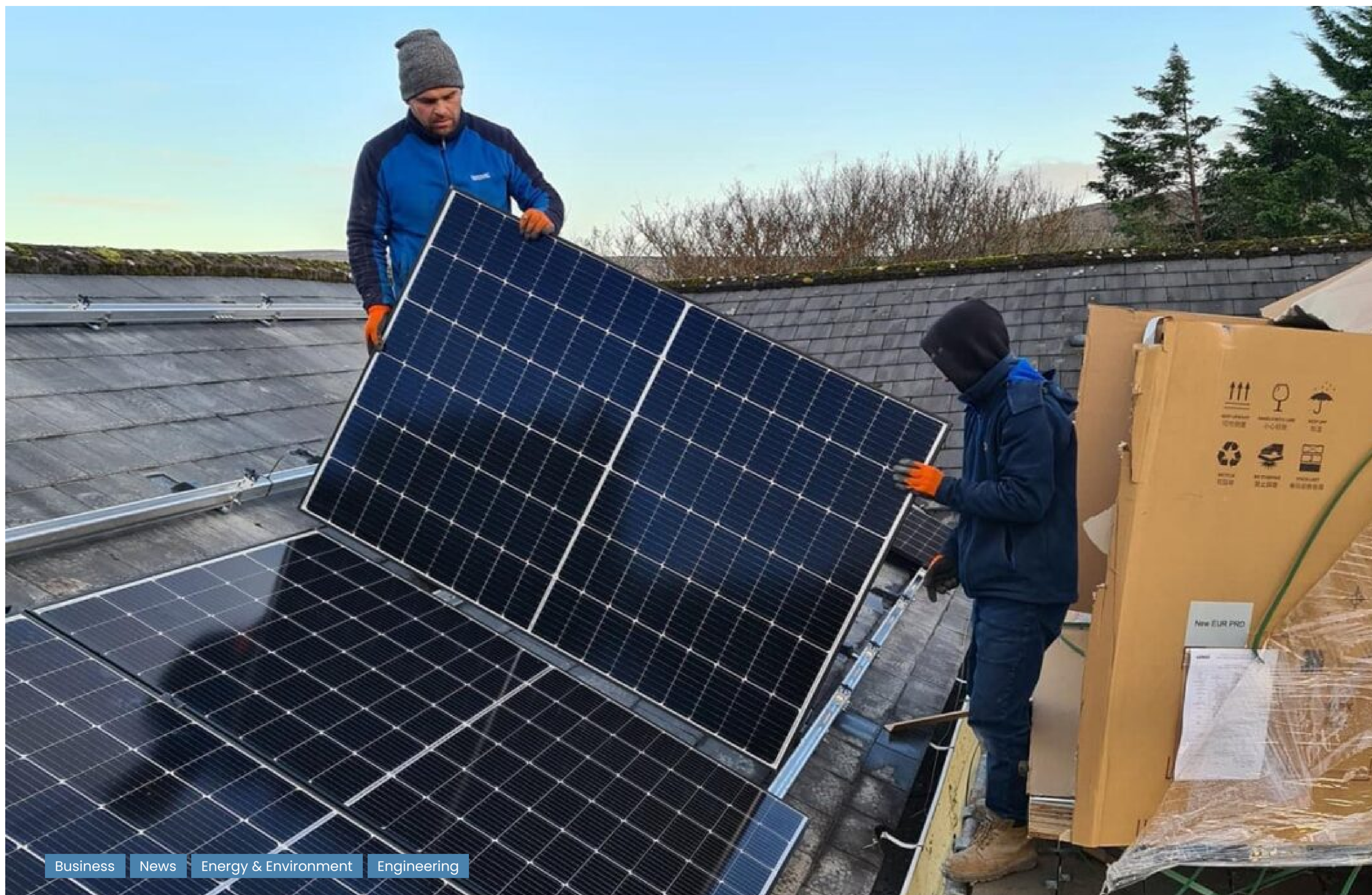
Solar panels being installed at Gregans Castle Hotel
